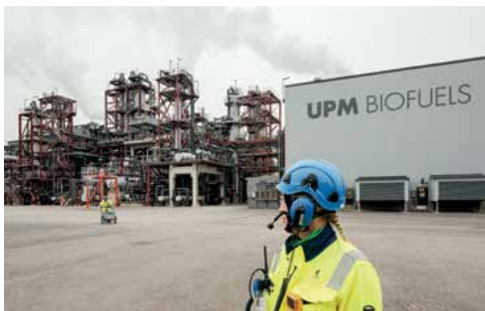
UPM Lappeenranta Biorefinery in Finland produces residue-based advanced biofuels (renewable diesel and naphtha)
